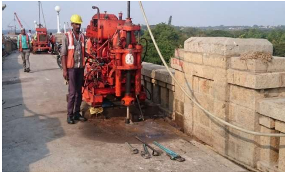
DRILLING & GROUTING WORKS IN PROGRESS
