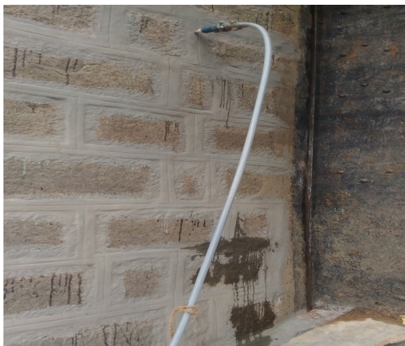
NOZZLE INSTALLED IN THE PIER PORTION
