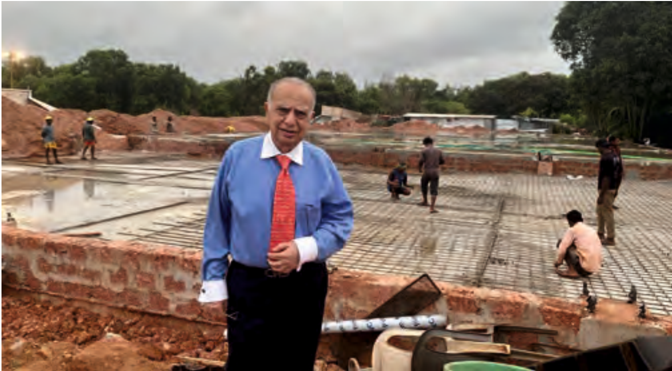
Progress on the new proposed Banquet Hall.
